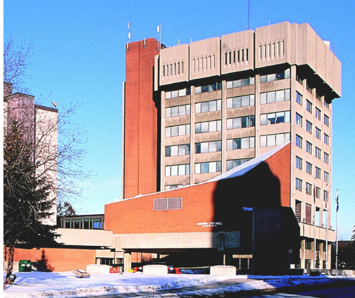
City of Oshawa Civic Administration Complex
